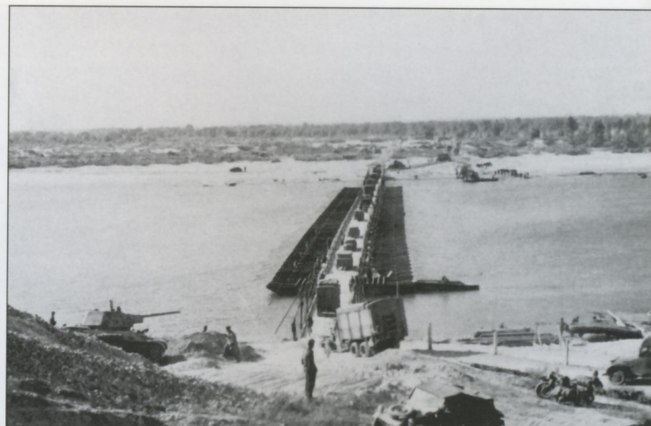
A rare opportunity to see vehicles crossing the Don during the 2. Panzer-Division's advance on the Volga in late August. These three photographs taken in sequence show the type of construction which was built by the divisional Pionier-Bataillon. A number of cross-country Horch cars can be seen crossing along with Opel "Blitz" trucks, halftrack personnel carriers, and other vehicles. In one of the photographs a captured Soviet T-34 tank can be seen to the left of the bridge's access. A white Balkenkreuz has been painted on the turret's side.
