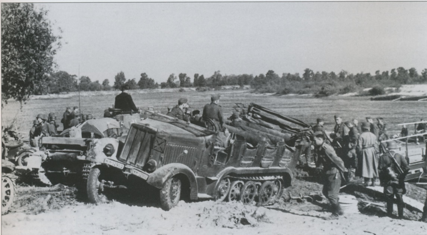
Early the following morning on 23 August a battalion of 2. Panzer-Regiment, reinforced with Panzergrenadier companies, advanced forward from the Don River towards the Volga. Here a 12-ton Sd.Kfz.8 halftrack has crossed the Don over a pontoon and trestle bridge.
